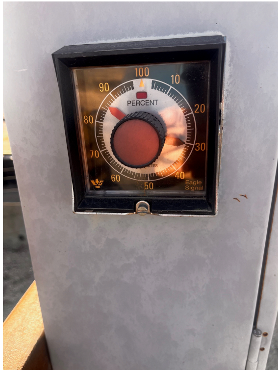
The percent timer controls the well based on a 15 minute clock
